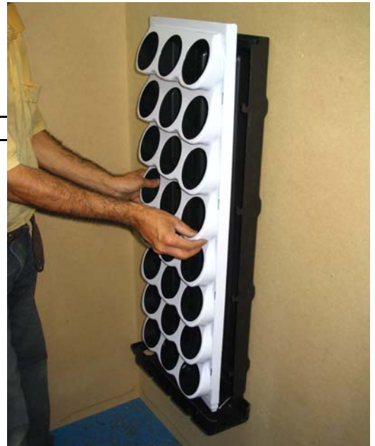
Fix the 24-hole culture support (white) on the small hooks of the back support (black) created for this.
